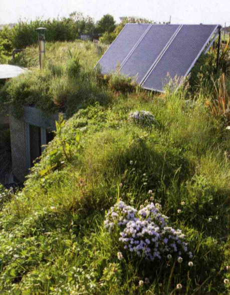
ABOVE The Harralls' water is heated by the solar panels on their roof, and although Jerry and Kay put in electric underfloor heating, the house is so well insulated they've only used it briefly on the coldest of days
